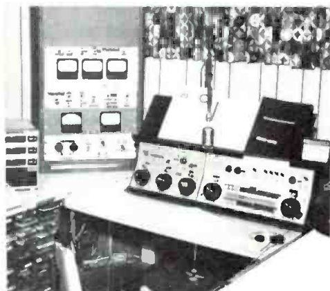
Fig. 4 AM control room with AM remote control and switching unit at center. The AM transmitter remained in the old station facility.
